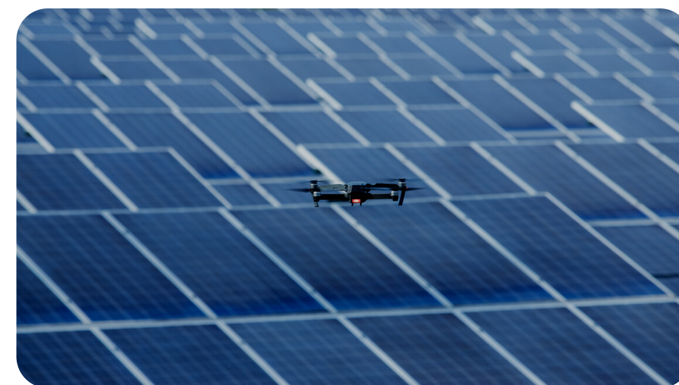
Solar Panels Inspection
